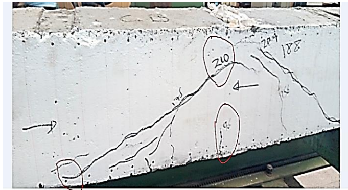
Figure 4-2 control beam at failure
