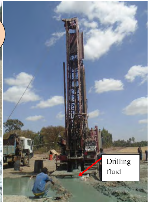
Plate 5.5 well drilling in Teji which affects nearby shallow wells dry
