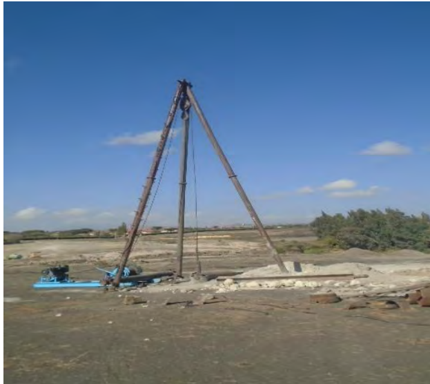
Plate 5.9 Cable tool well drilling near Mojo River
