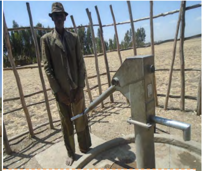
Plate 5.10 Hand pump well with no observation well in Becho area
