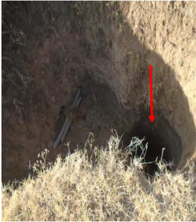
Plate 5.15 Dried Hand dug well in dry season around Holleta area
