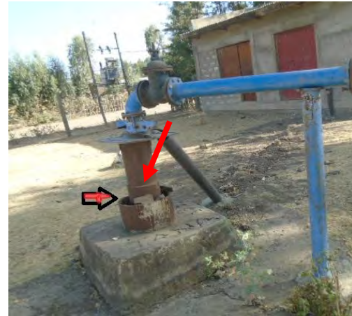
Plate 5.3 Opened annular space in Asgori production well
