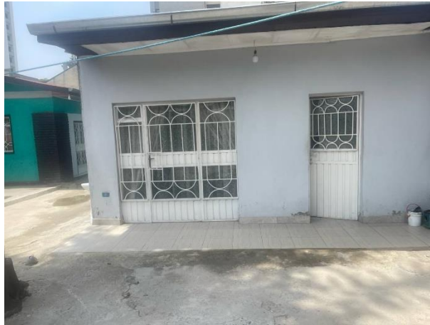
Figure 4:- Existing G+0 residential building
