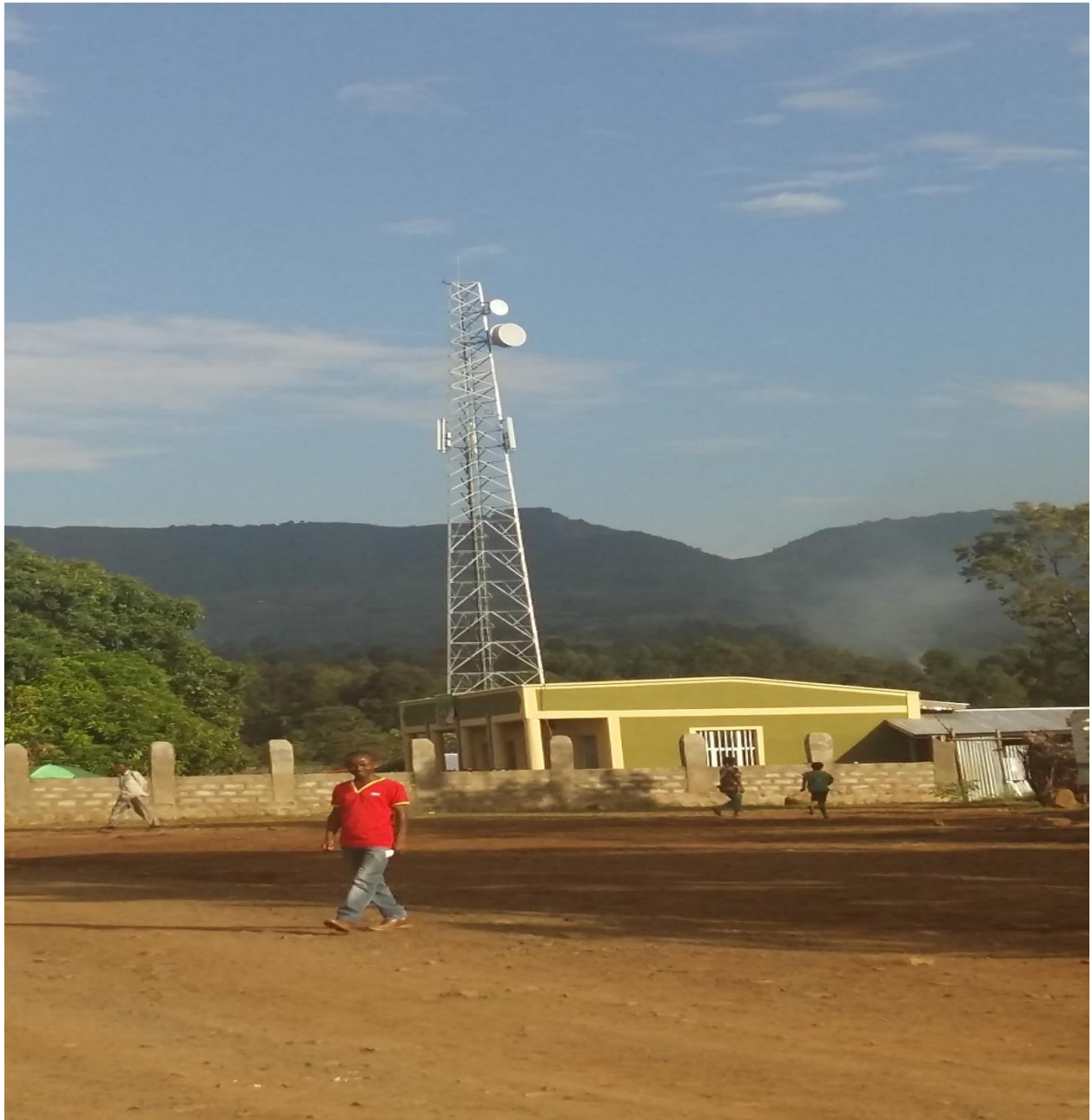
Figure .2 Tele tower & office
