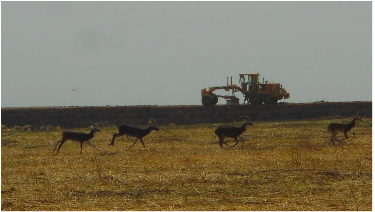
Appendix 9. Road construction in the GNP (Nhial Tuach, 2018).
