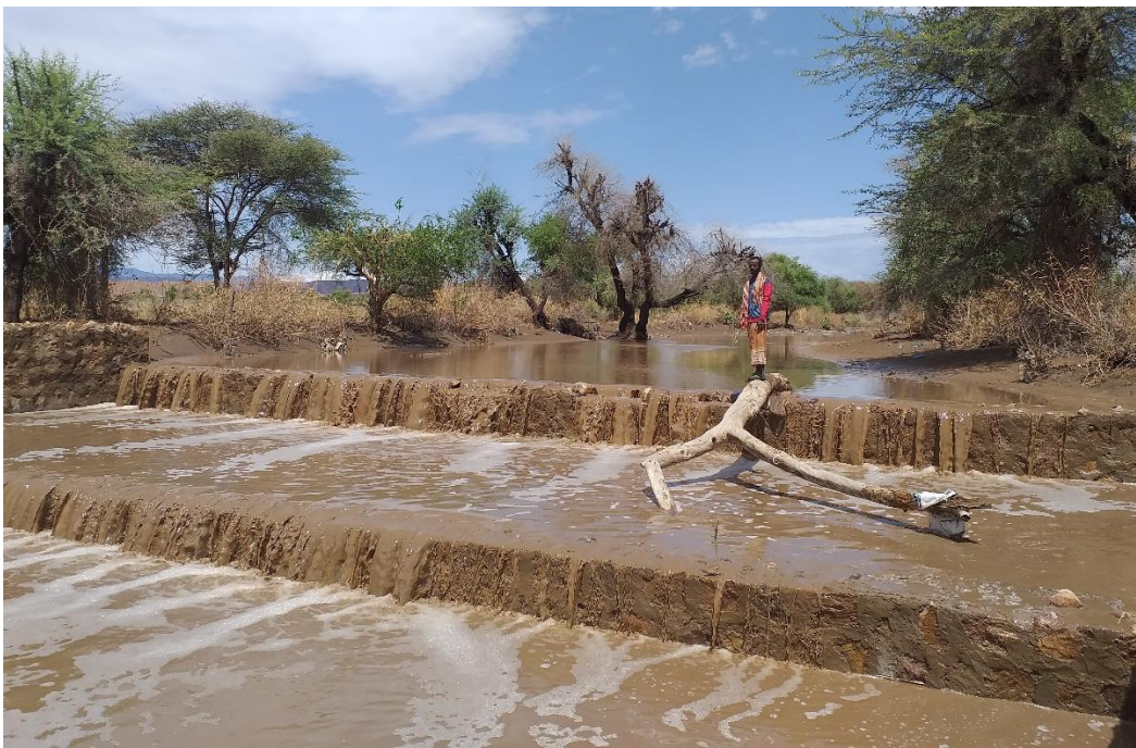
Figure 9: Water-spreading Weirs in Chifra
