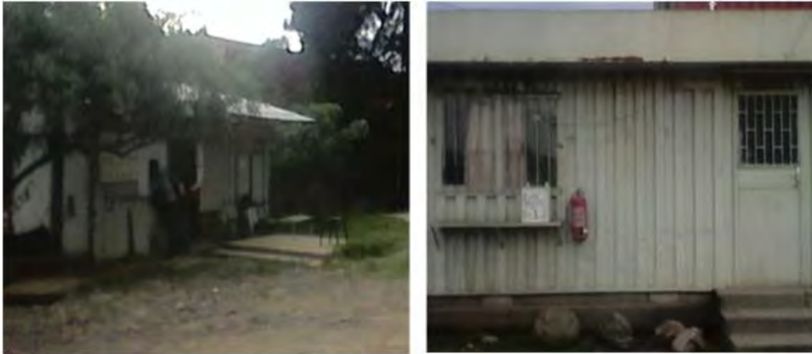
Figure 4. Office facilities for dry port employees
