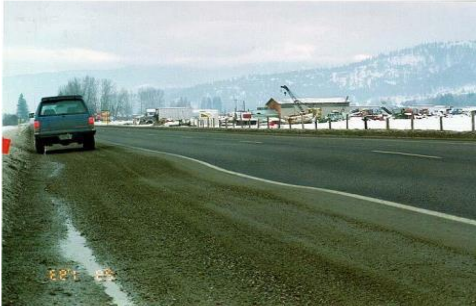
Figure 2.8 Depressions Type Surface Deformation in Flexible Pavement
