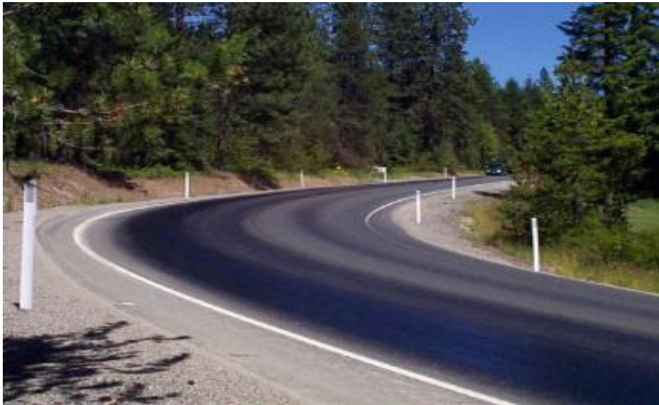
Figure 2.11 Bleeding Type Surface Defects in Flexible Pavement
