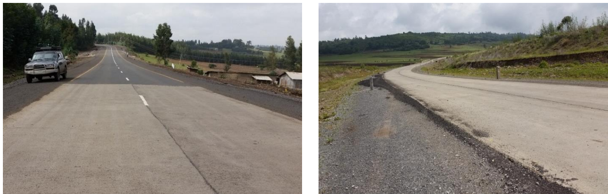
Figure 2.7. Chanco Derba Becho road project; beginning of the concrete rigid pavement (left) and somewhere in middle section of the concrete road (right)
