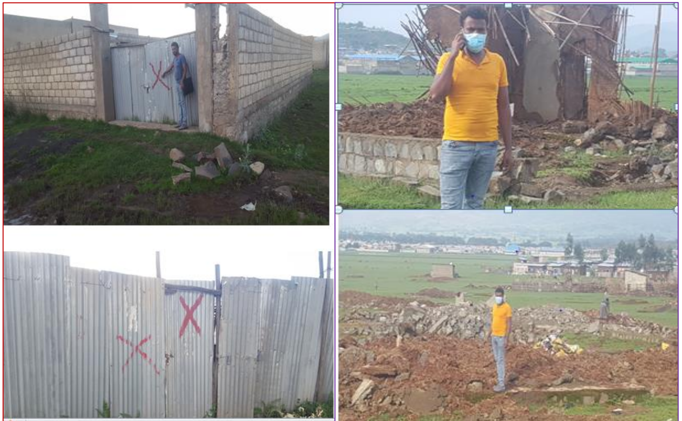
Figure: 4.7-informal house identifies for demolishing and demolished in Sululta Town
