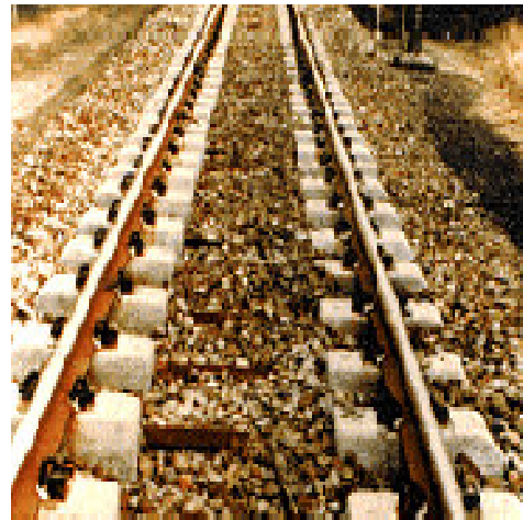
(b) Twin-block sleepers
