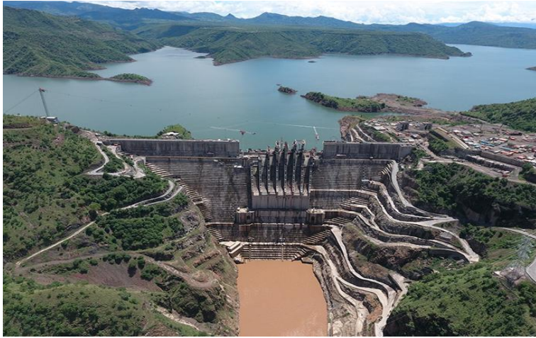
Image2. Topographic view of the project site
