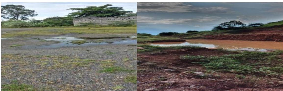
Image 3, some parts of the environment damaged by the construction activities
