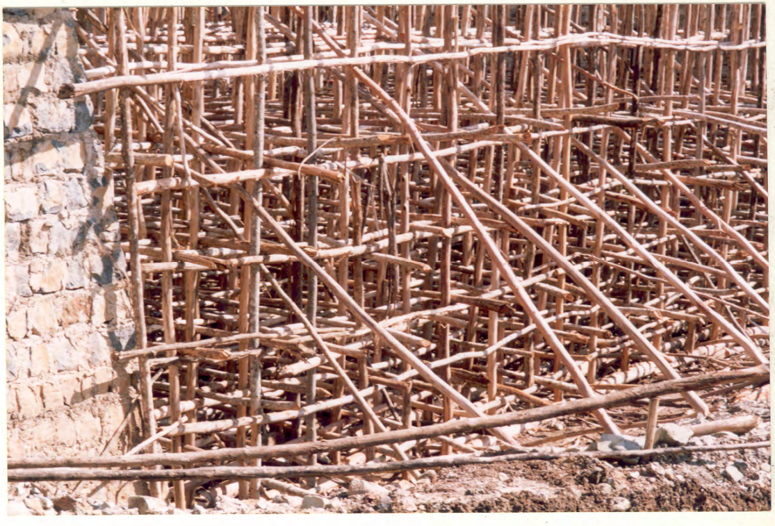
Figure 5.6 Completed false work for Kilkile Bridge
