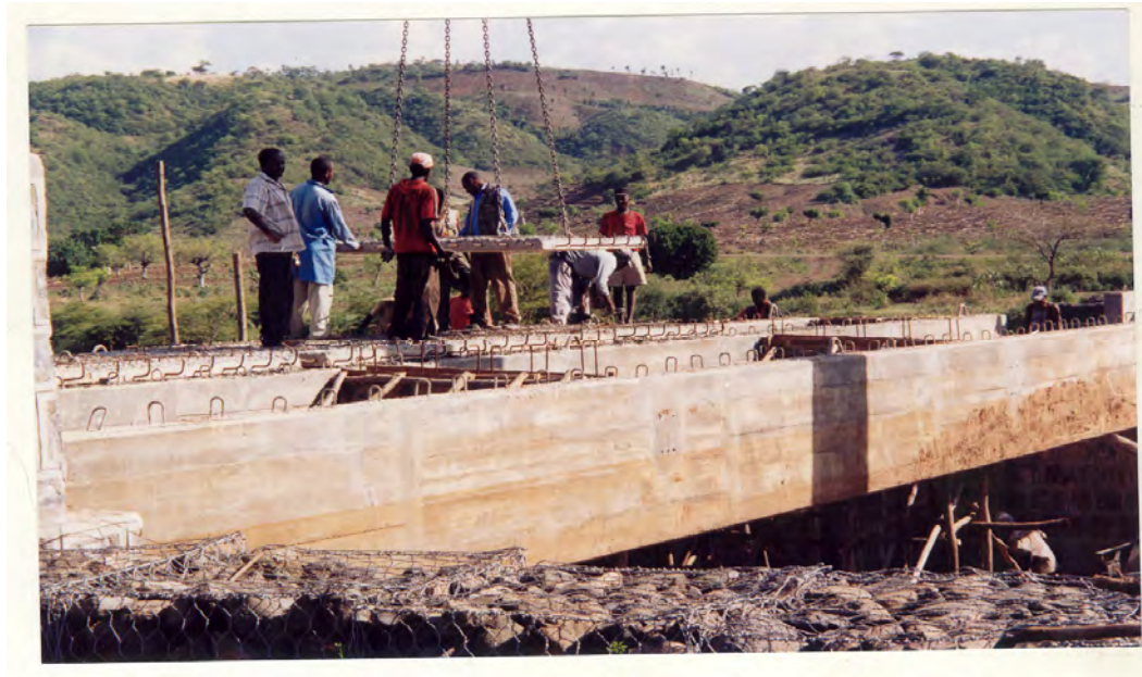
Figure 5.9 Erection of precast part of the deck
