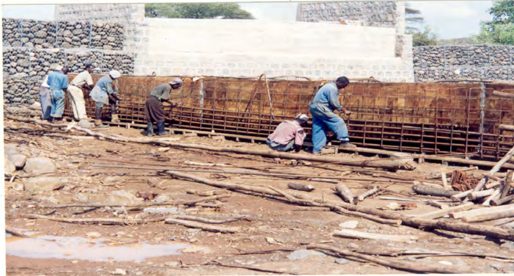
Figure 5.7 Placing of reinforcement for precast girder
