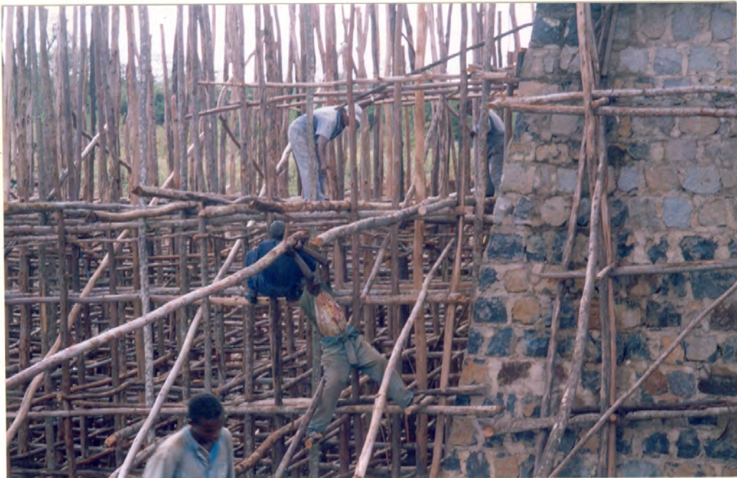
Figure 5.5 False works under construction for precast bridge at Kilkile River
