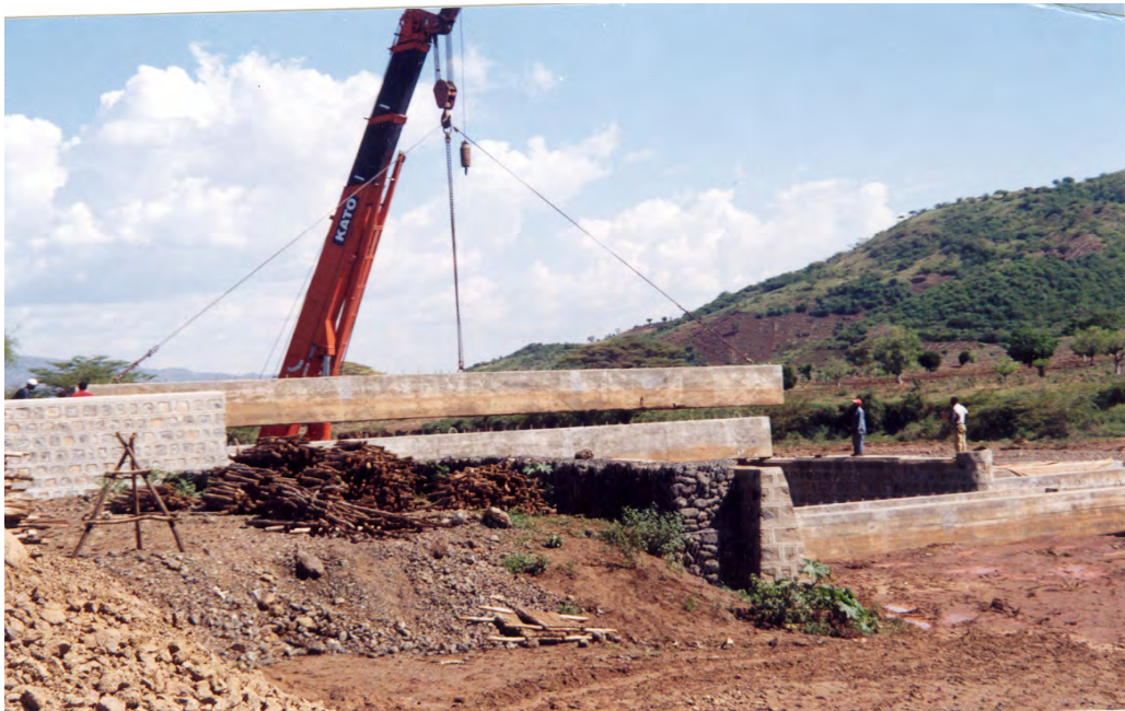
Figure 5.8 Erection of precast girder
