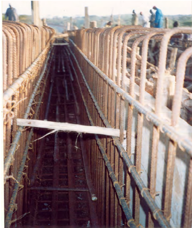
Figure 5.3 Reinforcement arrangements for girder shear and moment
