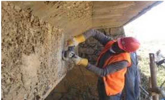
Plate 5.3.2a: Saw cut and chipping
