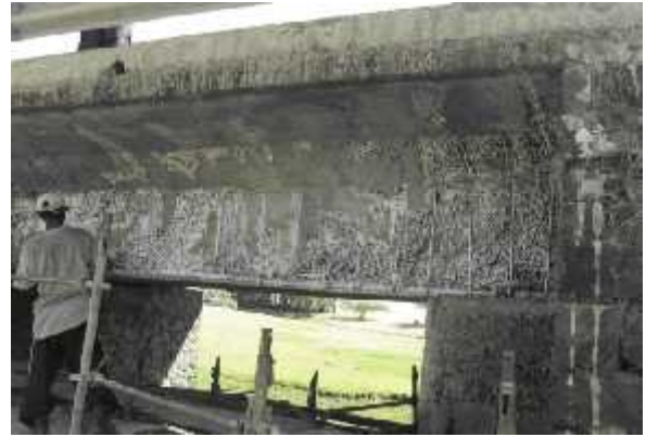
Plate 5.3.1b: NitoBond application
