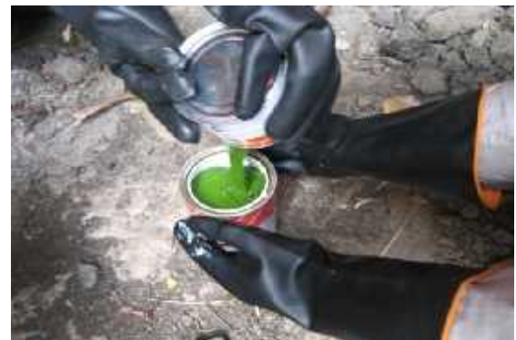
Plate 5.2.1b: Pouring hardener in to base
