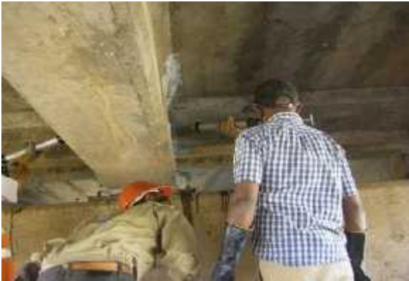
Plate 5.2.4i: Injecting Nitofill EPLV or CONCRESSIVE 1414
