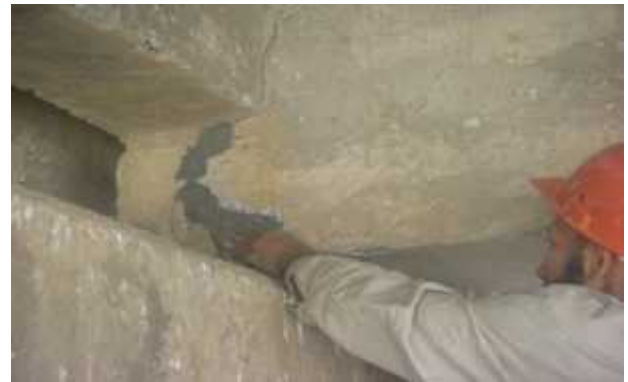
Plate 5.2.4b: Sealing the crack with EMACO S88CT
