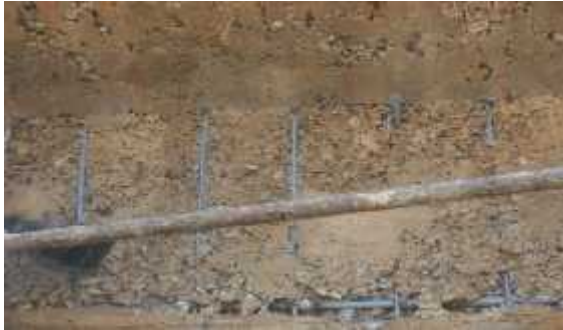
Plate 5.3.2c: Cleaning by jet water and painting anti rust
