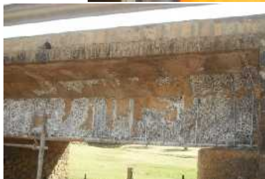
Plate 5.3.2d: Applying NitoBond
