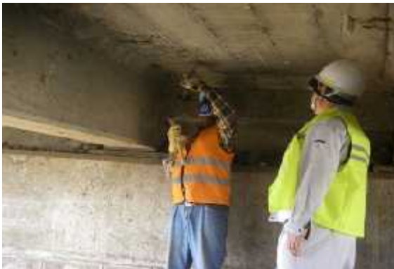
Plate 5.2.2c: Chipping or removing the deteriorated concrete
