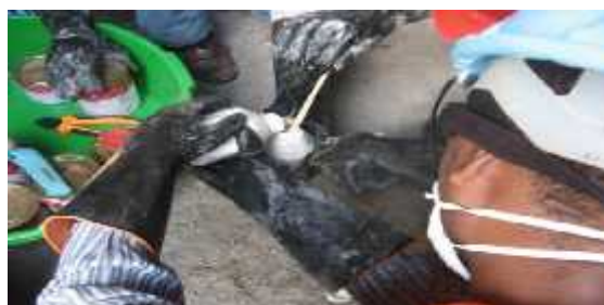
Plate 5.2.1i: Nitofill (mixing)
