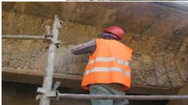
Plate 5.3.2a: Saw cut and chipping
