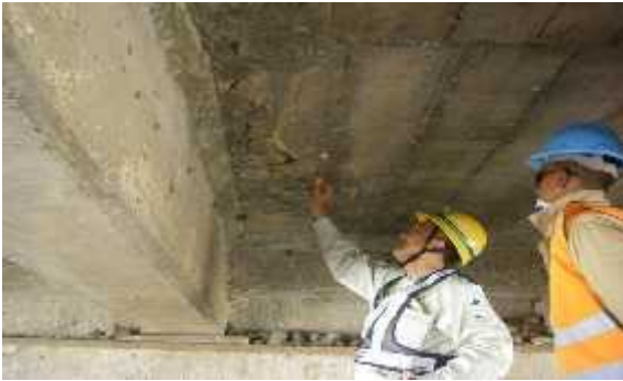
Plate 5.2.2a: Honeycombed surface
