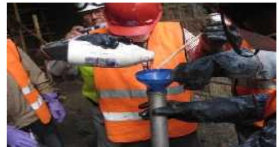
Plate 5.2.1j: Concresive (mixing)
