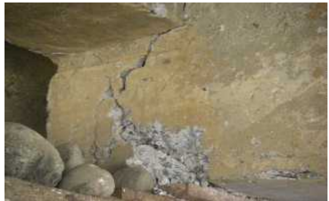
Plate 2.2.1b: Shear crack
