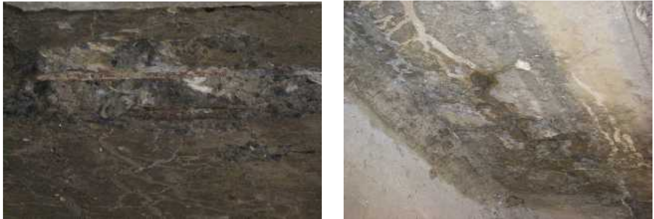
Plate 2.2.4: Surface scaling
