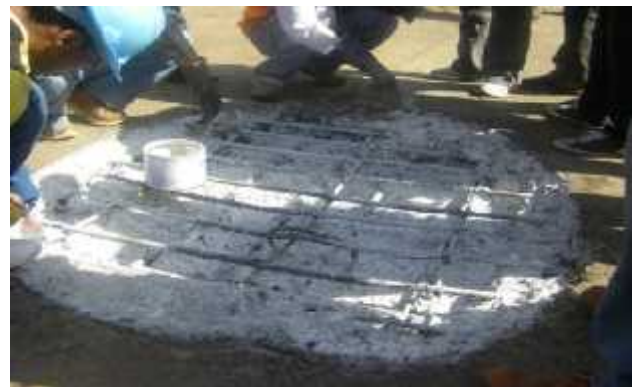
Plate 5.2.3c: Applying Bonding Agent Concretive 1414
