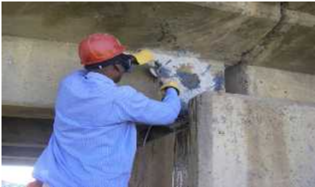
Plate 5.2.4j: Cutting the pipes with grinder
