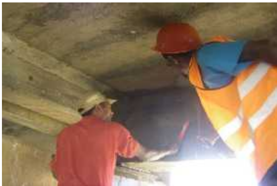
Plate 5.2.4a: Cleaning with water jet
