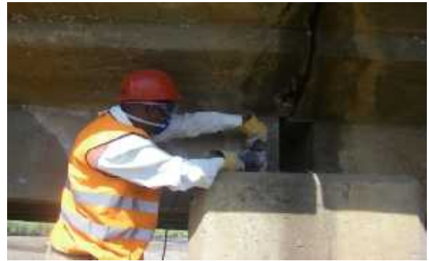
Plate 5.2.4d: Cleaning using grinder
