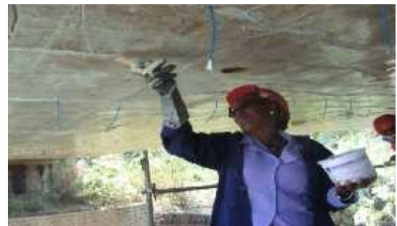
Plate 5.3.1h: Concresive 2200 application
