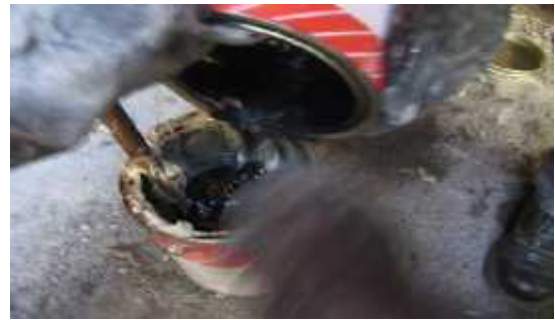
Plate 5.2.1l: Nitomortar (pouring)
