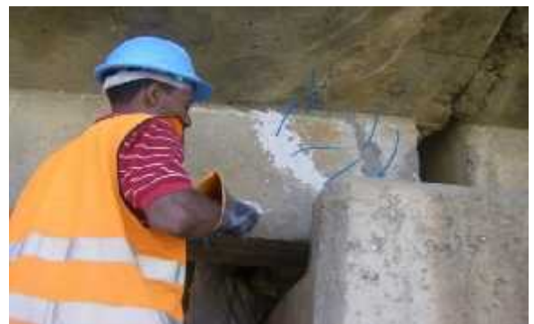
Plate 5.2.4h: Sealing the crack and holes with NITOMORTAR
