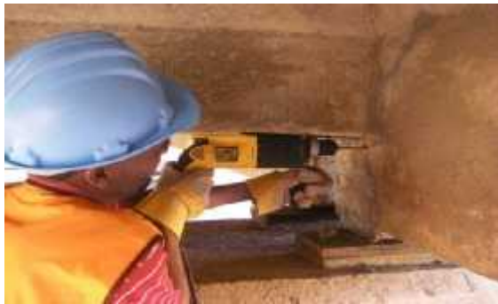
5.2.4e: Drilling holes diameter of 6mm at 15 cm spacing
