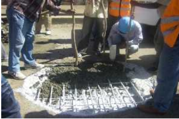
Plate 5.2.3h: Placing concrete treated with Fiber (Rhofiber)
