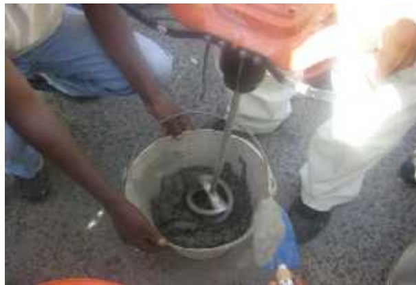
Plate 5.2.3g: Mixing concrete with fiber (Rhofiber)
