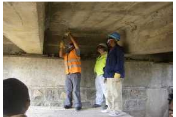
Plate 5.2.2c: Chipping or removing the deteriorated concrete
