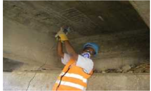
Plate 5.2.2b: Cut the defect with grinder to make small squares with 5cm sides
