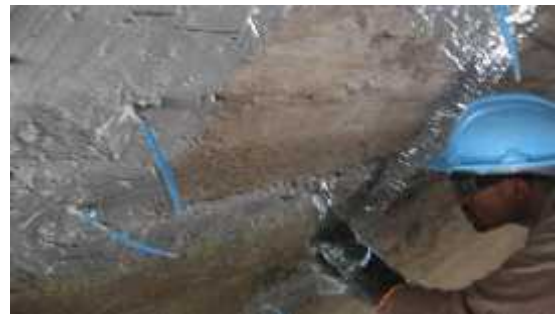
Plate 5.2.1n: Nitomortar application)
