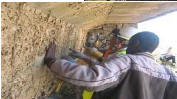
Plate 5.3.2b: Grinding and removing of corrosion
