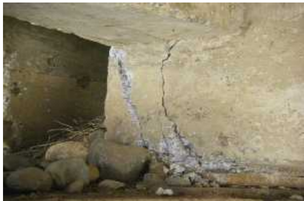
Plate 2.2.1b: Shear crack
