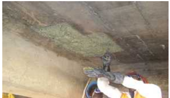
Plate 5.2.2g: Applying Bonding Agent (Nitobond EP)
