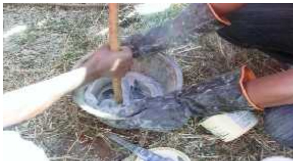
Plate 5.3.1g: Concresive 2200 (mixing)
