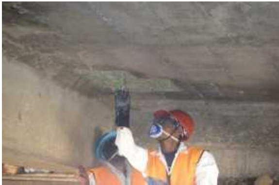
Plate 5.2.2e: Applying anti-rust paint
