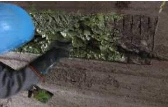
Plate 5.2.1e: Application of NitoBond
