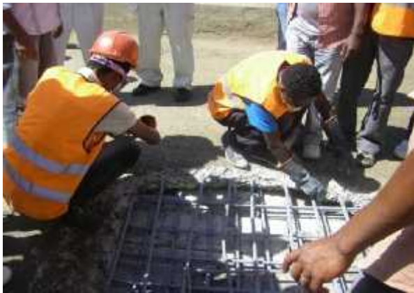
Plate 5.2.3f: Applying Bonding Agent Nitobond
