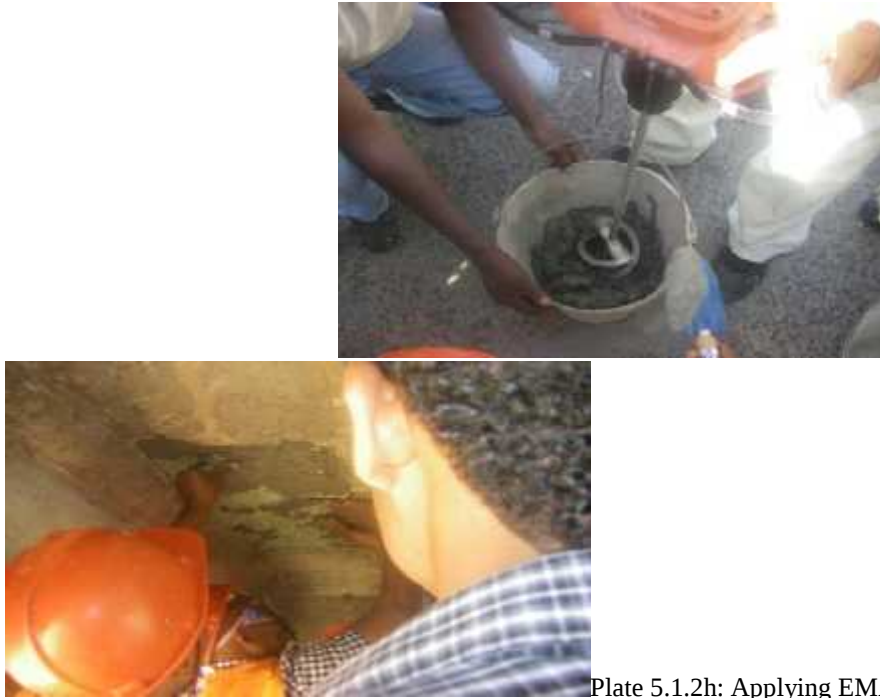
Plate 5.1.2h: Applying EMACO S88CT placing and curing
