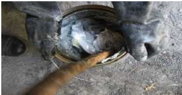
Plate 5.2.1m: Nitomortar (stiring)
