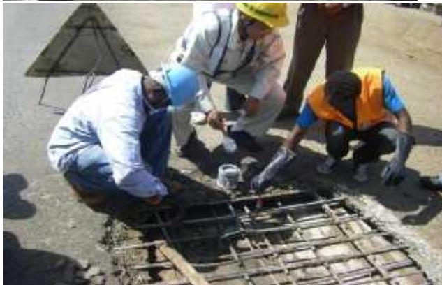
Plate 5.2.3a: Remove the deteriorated concrete around the hole with hammer, construct the formwork (soffit), Cleaning with water jet and applying anti-rust paint
