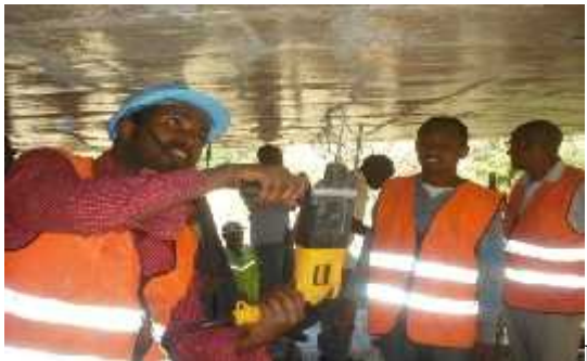
Plate 5.3.3b: Drilling injection hole
