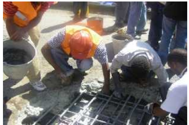
Plate 5.2.3f: Applying Bonding Agent Nitobond
