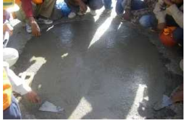
Plate 5.2.3i: Finished repaired concrete
