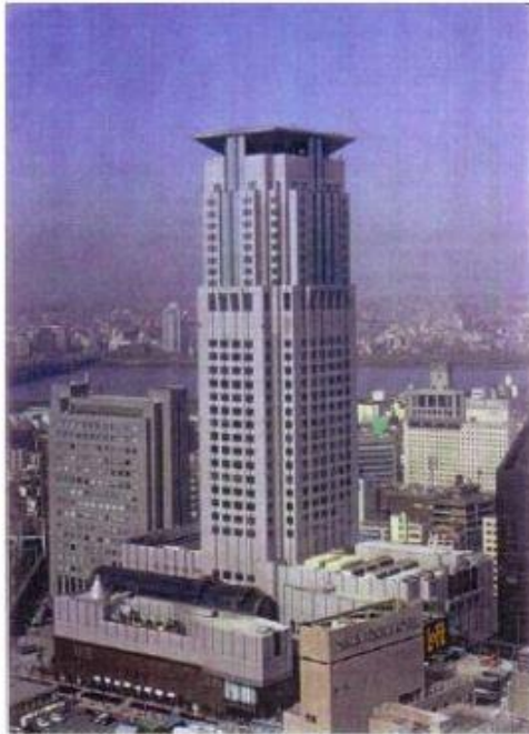
Figure 1.9 Active Mass Damper Using a Rooftop Heliport in the Applause Tower, Osaka, Japan
