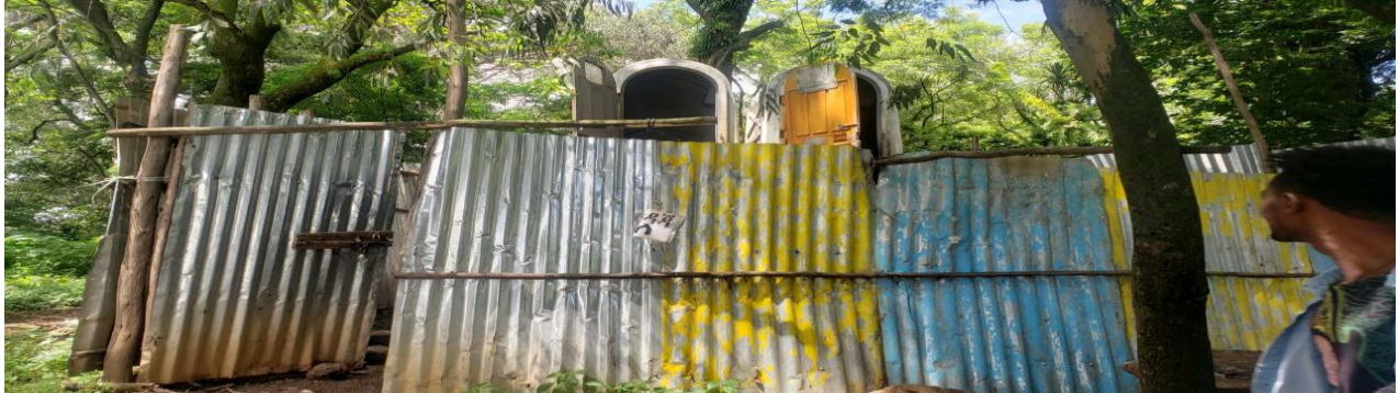
Figure 4. 4: The only wash room on the Lake Tana region
