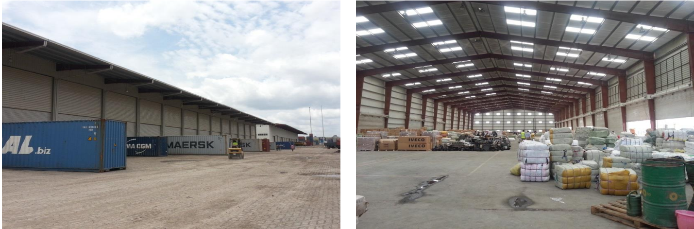
Figure 11: Warehouses at Mojo dry port (Exterior and Interior)
