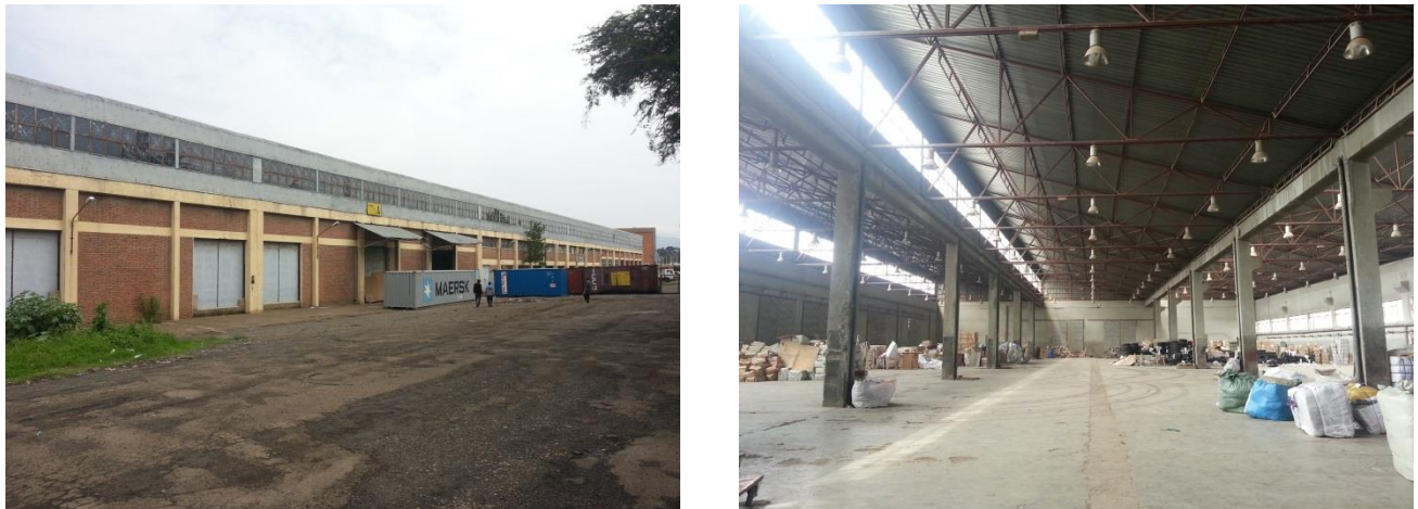
Figure 14: Kality customs examination warehouse
