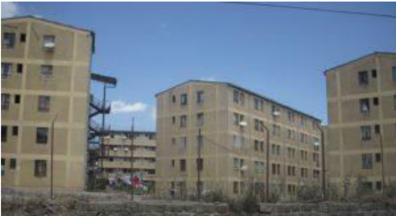
Fig 1. Partial View of Summit Condominium Site
