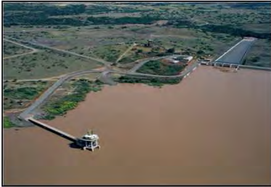
Figure 3-5 Photograph view of Gibe I dam and reservoir It is possible to see intake tower and the spillway chute.
