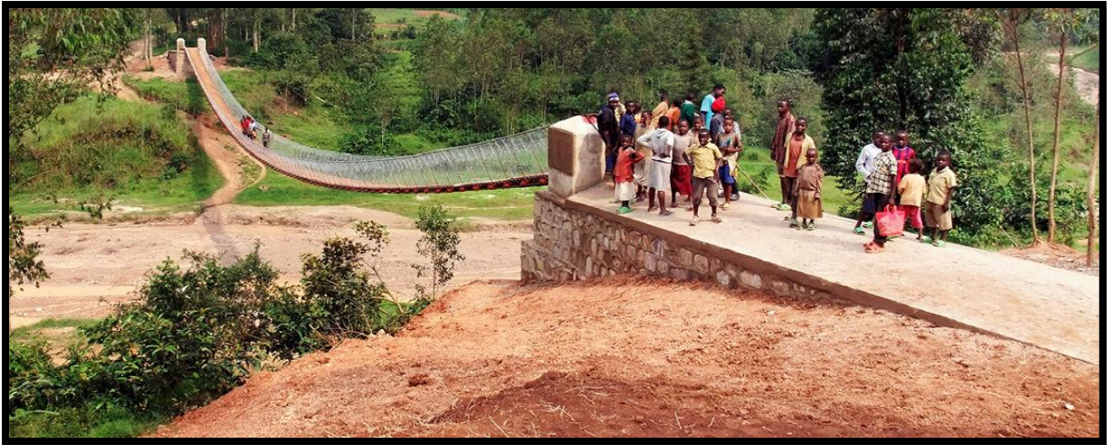
Figure 1.2 Typical Suspended Footbridge [1].
