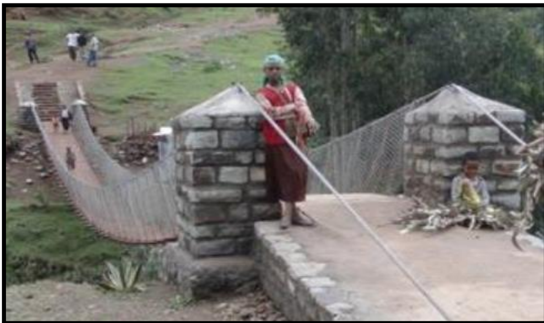
Figure 3.1 Basic case study pedestrian cable suspended bridge
