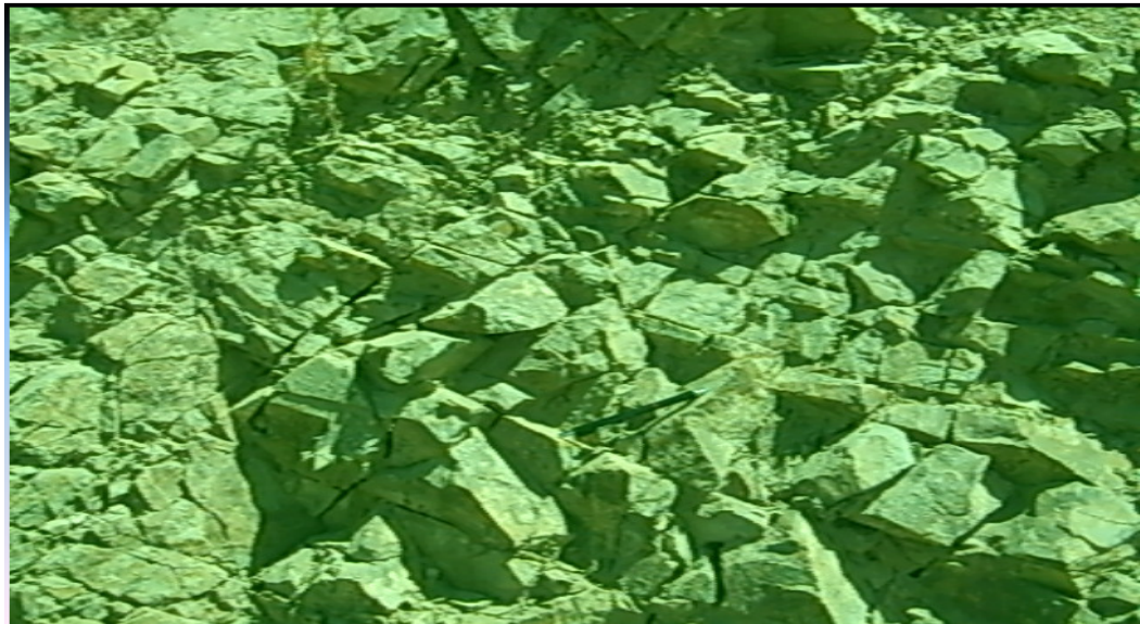
Figure 3.1: Rhyolite that shows NNE-SSW and ENE-WSW trending set of joints (Pen is oriented to the East) adopted from ORDA, 2008.
