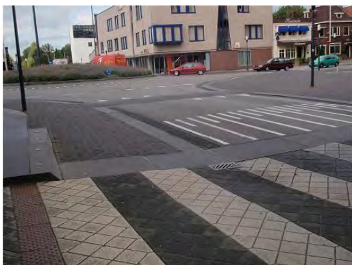
Figure 16. Laweiplein-roundabout entry ramp (Source: Hamilton-Baillie, 2005)
