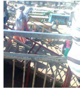
2 Stair led to Megenagna terminal
