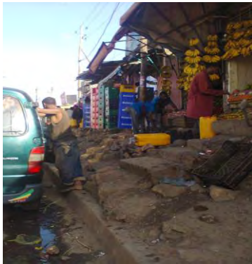
3 Poor condition shops
