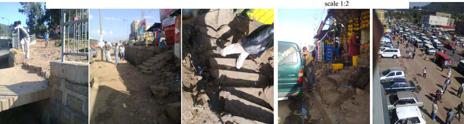
Figure 21. Connectivity of roundabout with surrounding and the connecting elements (source; Addis Ababa structural road network map and edited based on survey and photo taken by; Senait Mohammed, 2006 )
