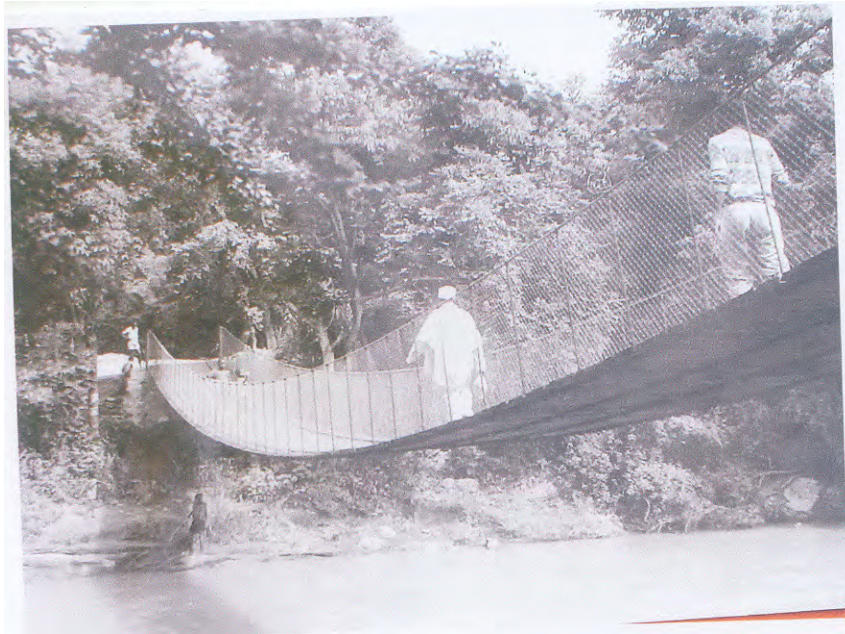
Figure 3 Suspended cable bridge at Gambela.
