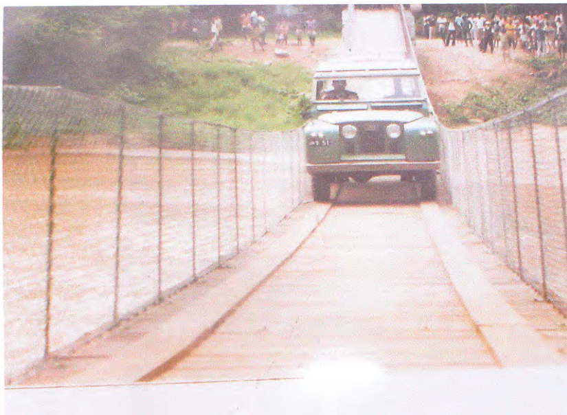
Figure 2 Suspended cable bridge at Gambela.
