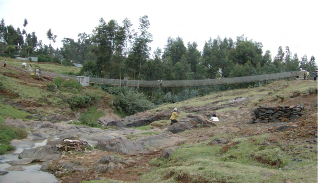
Figure 1 Suspended cable bridge at Kolfe Keraneyo(9).
