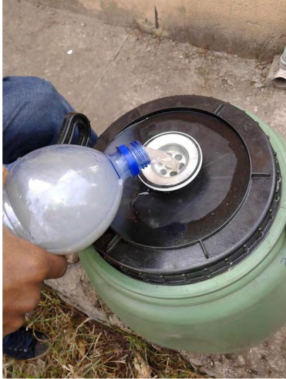
Add the collected untreated grey water until it fills the barrel
