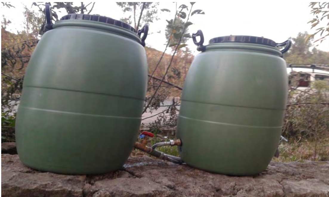
Set and install the two barrel with flexible steel pipe
