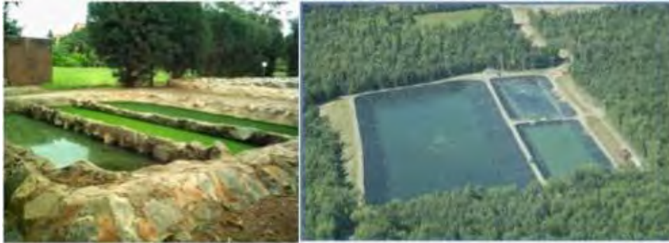
Figure 12: Waste Stabilization Ponds (WOC, 2013)
