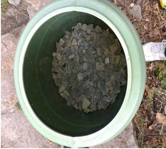
Add the gravel at the bottom of the first barrel
