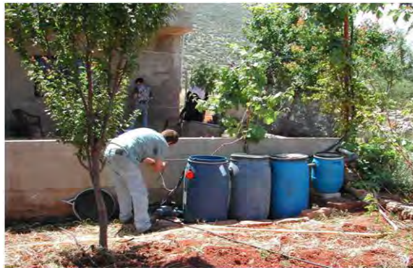
Figure 17: Four-Barrel Treatment Units (AL-BEIRUTI, 2004)
