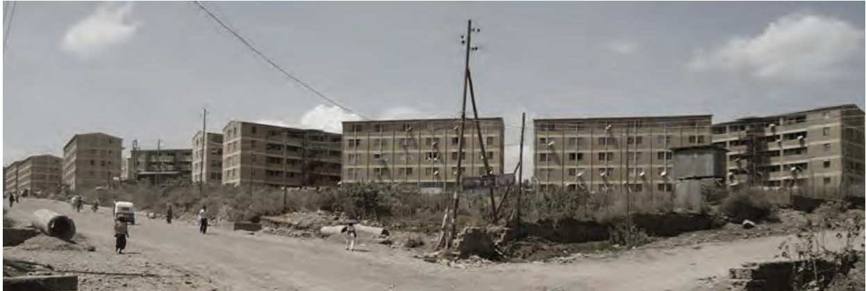
Figure 22. The view of the Repi I site from South.
