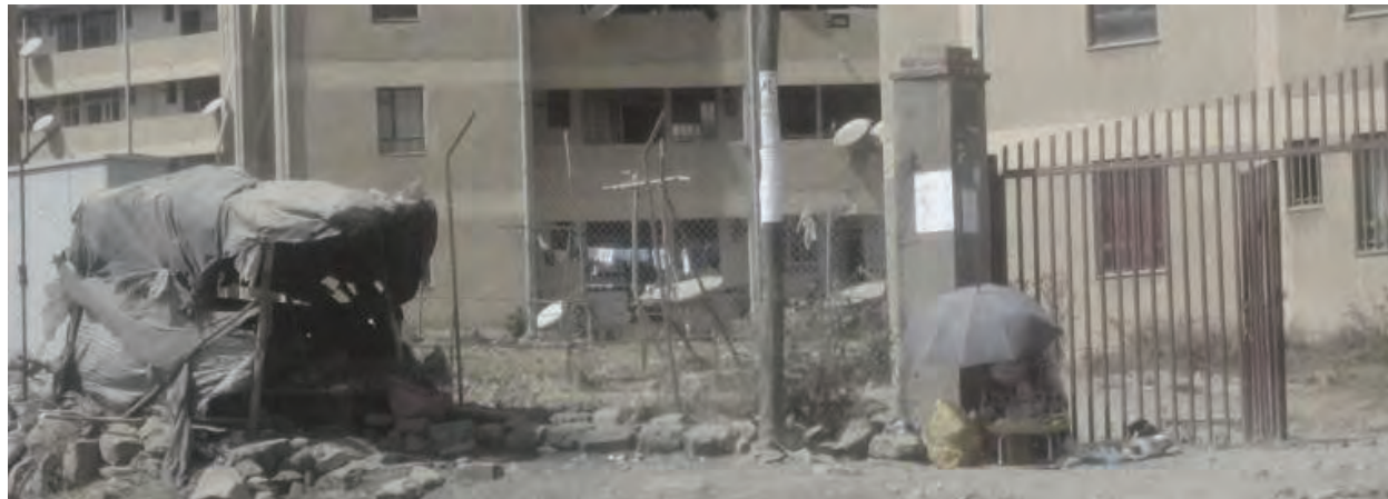
Figure 34. Two vendors in the main gate of Repi I site.
