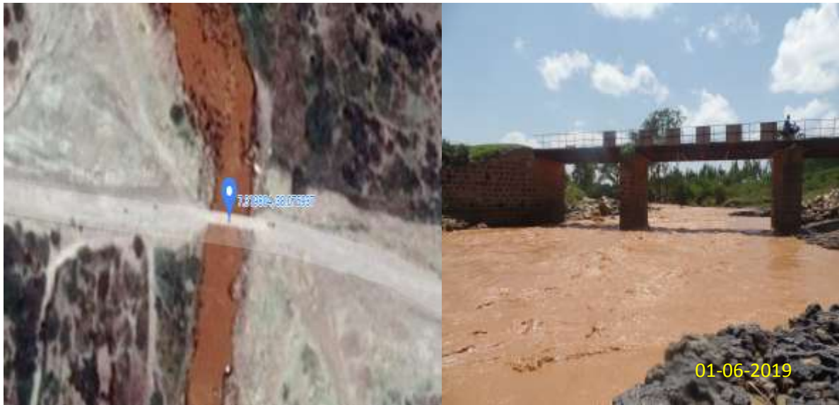
Figure 3.3: The Bilate River Bridge
