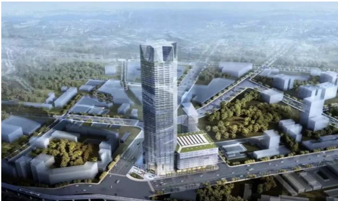
Figure 6. Future BOA Head Office
