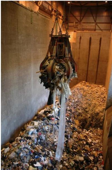
Figure 6 : A picture of a typical municipal solid waste bunker device
