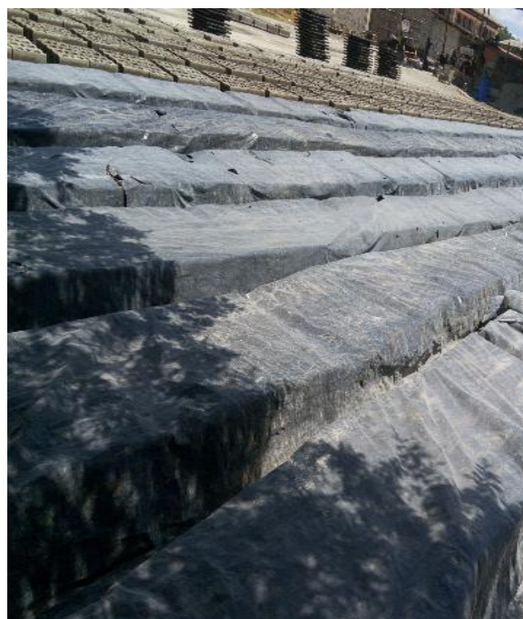
[f]: - curing by coveering with plastics
