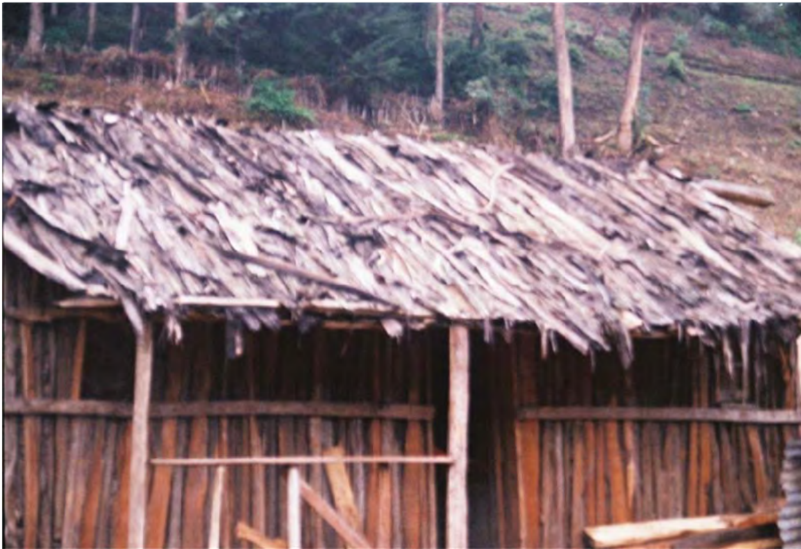
Plate 9: One of the local houses whose roof is made of the bark of Juniperus procera (Photo by Shambel Bantiwalu, 2009).
