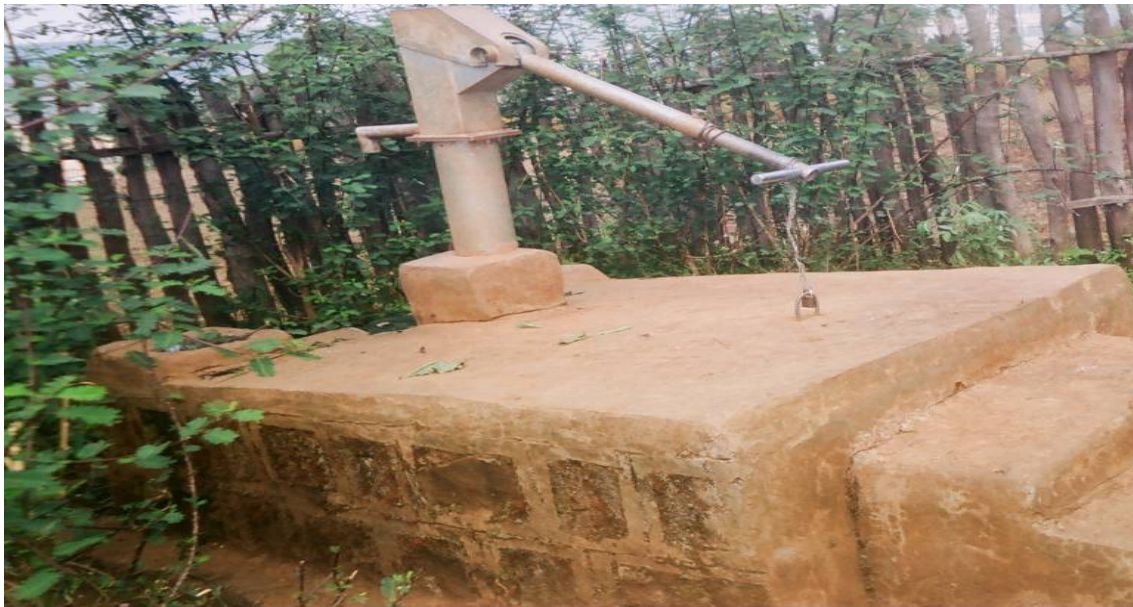
Photo 5.2: Non Functional Water Supply Schemes in Yewula (Yecholit village) because of polluted with iron minerals
