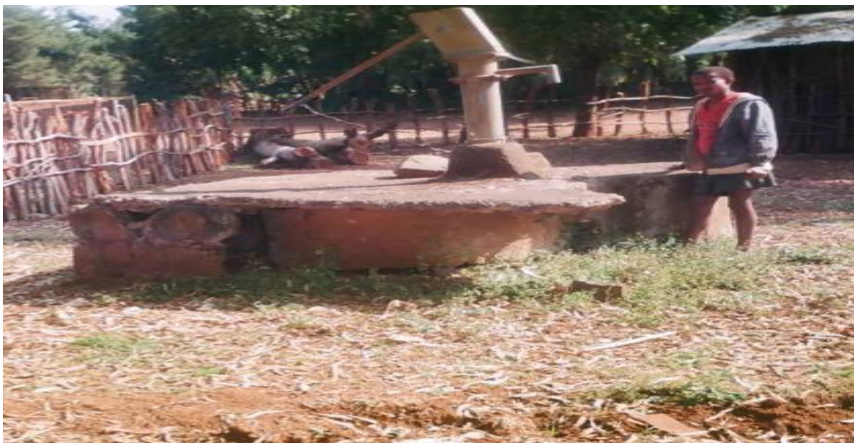
Photo 5.3: Non Functional Water Supply Schemes Because Of Poor Construction Quality in Sostu Deber Shelel in (Shelel- guilt) village)
