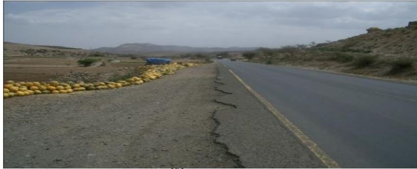
Figure 9. Edge Cracking [9]
