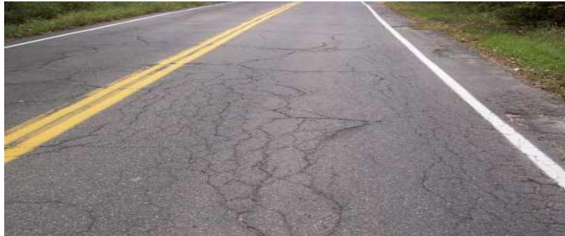
Figure 4. Alligator Cracking [8]
