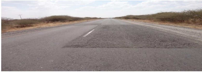
Figure 17. Patching (NET Consult Consulting Engineers and Architects Plc)
