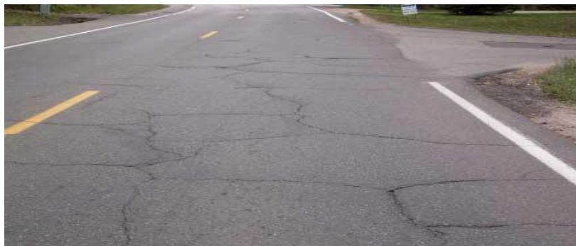
Figure 7. Block Cracking [8]
