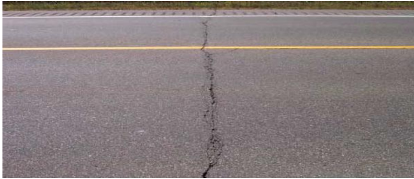
Figure 6. Transverse Cracking [8]
