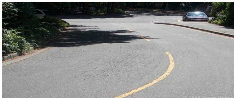
Figure 14. Depression ( www.pavementinteractive.org )
