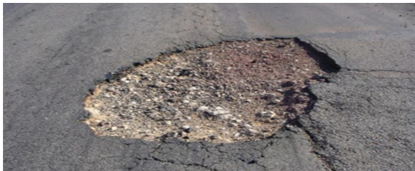
Figure 16. Potholes [10]
