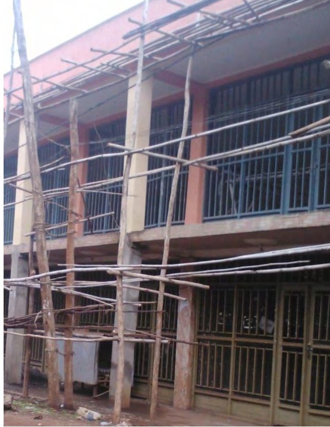
Figure 3-9: Bamboo-wood composite scaffolding system in Assosa Town
