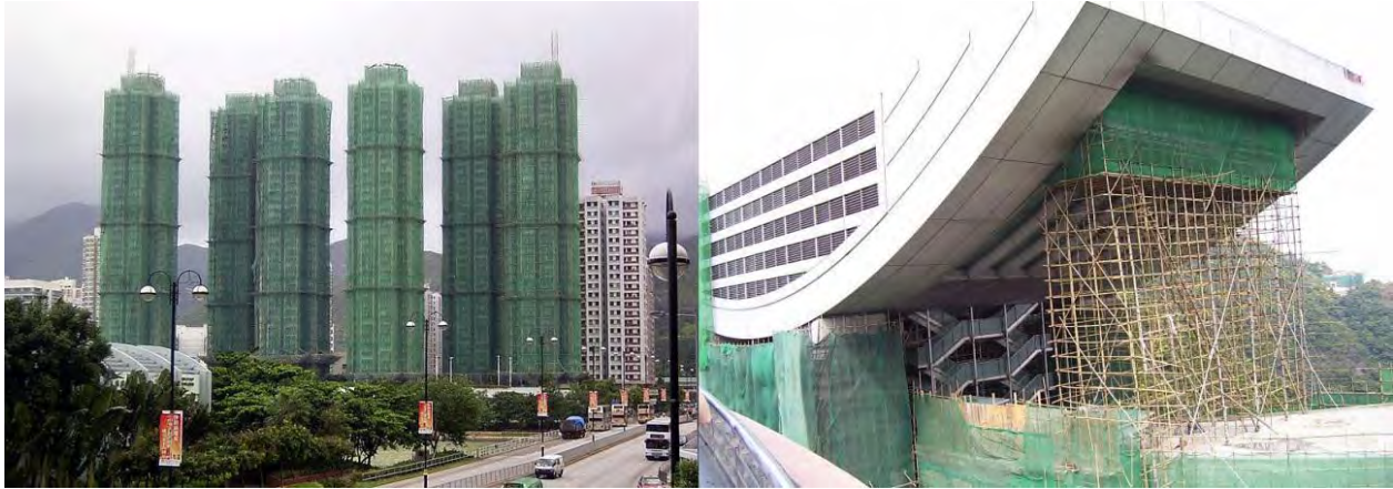
Figure 3-8 Bamboo high-rise scaffolding in Hong Kong, China (Source: Chan 2002)
