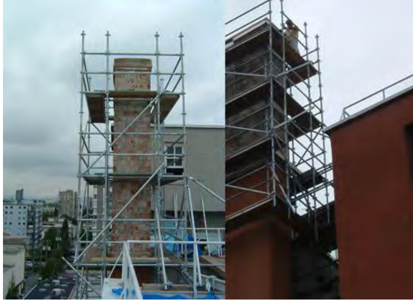
Figure 3-5: Cantilever or needle scaffolding (Source: WWW.hdwalls.xyz)
