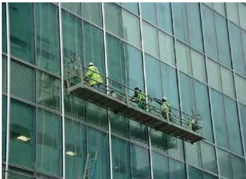
Figure 3-6: Suspended Scaffolding( Source: WWW.wti-scaffold.com)
