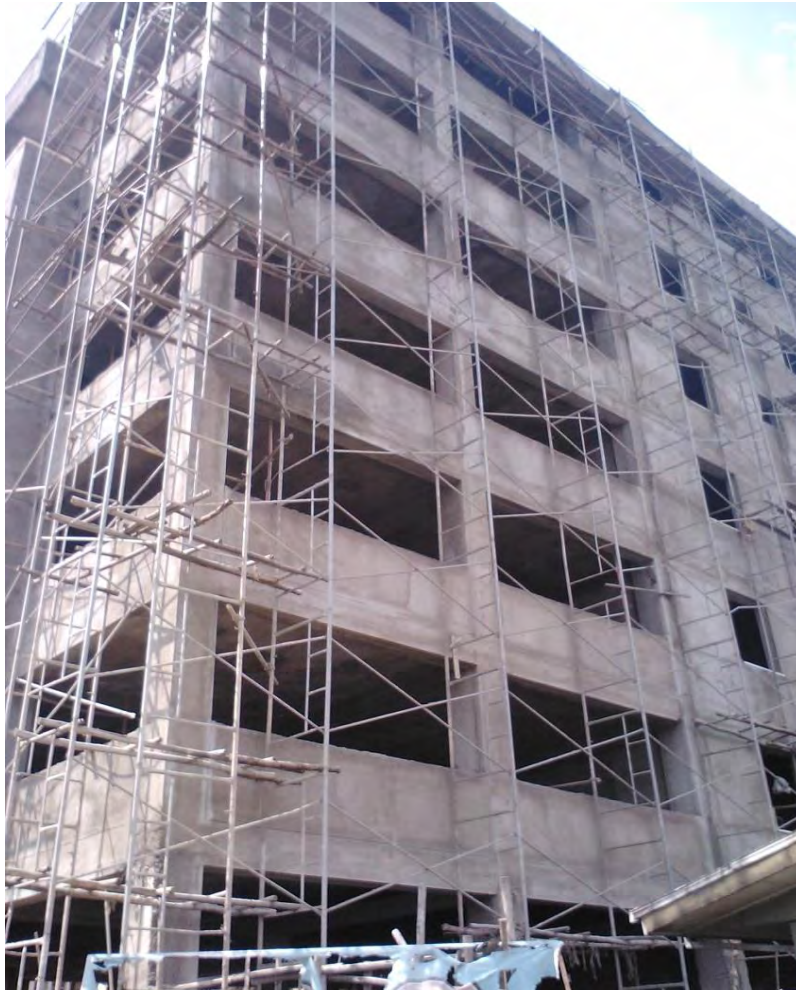
Figure 3-3: Double Scaffolding made of steel around Lagar area
