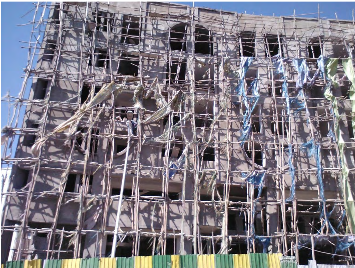
Figure 3-4: Wood Scaffold of Building around Arat Kilo
