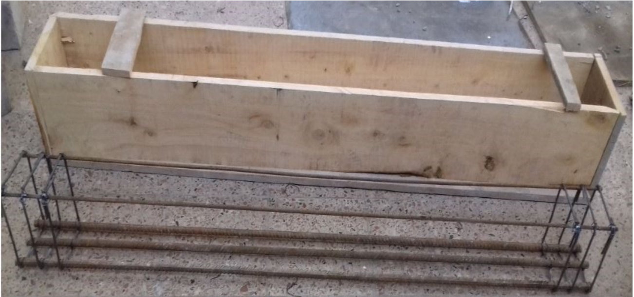
Figure 4:4: Reinforcement cage and formwork of the specimens
