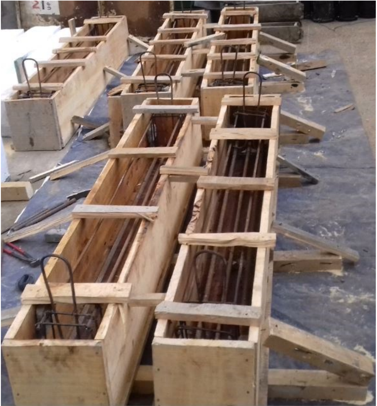
Figure 4:5: Reinforcement cage of specimens inside the formwork
