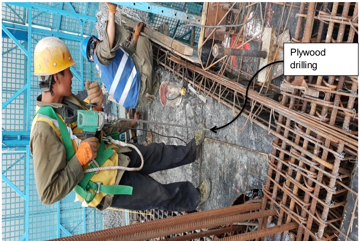
Figure 15 Plywood drilling machine for tying by treaded bar
