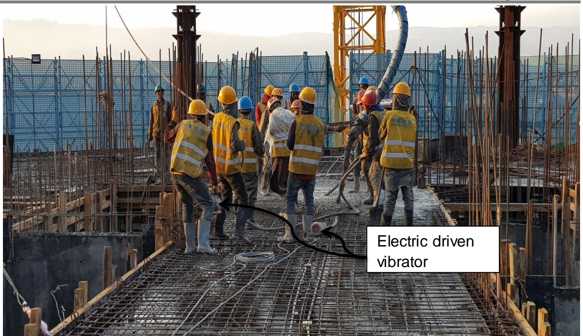
Figure 14 Concrete casting using vibrator which works with electric power
