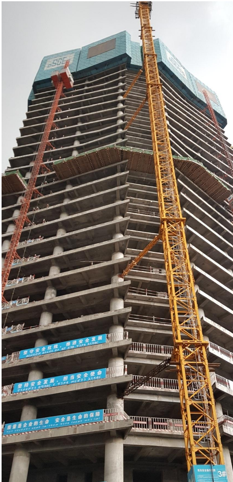
Figure 10 CBE office tower building under construction
