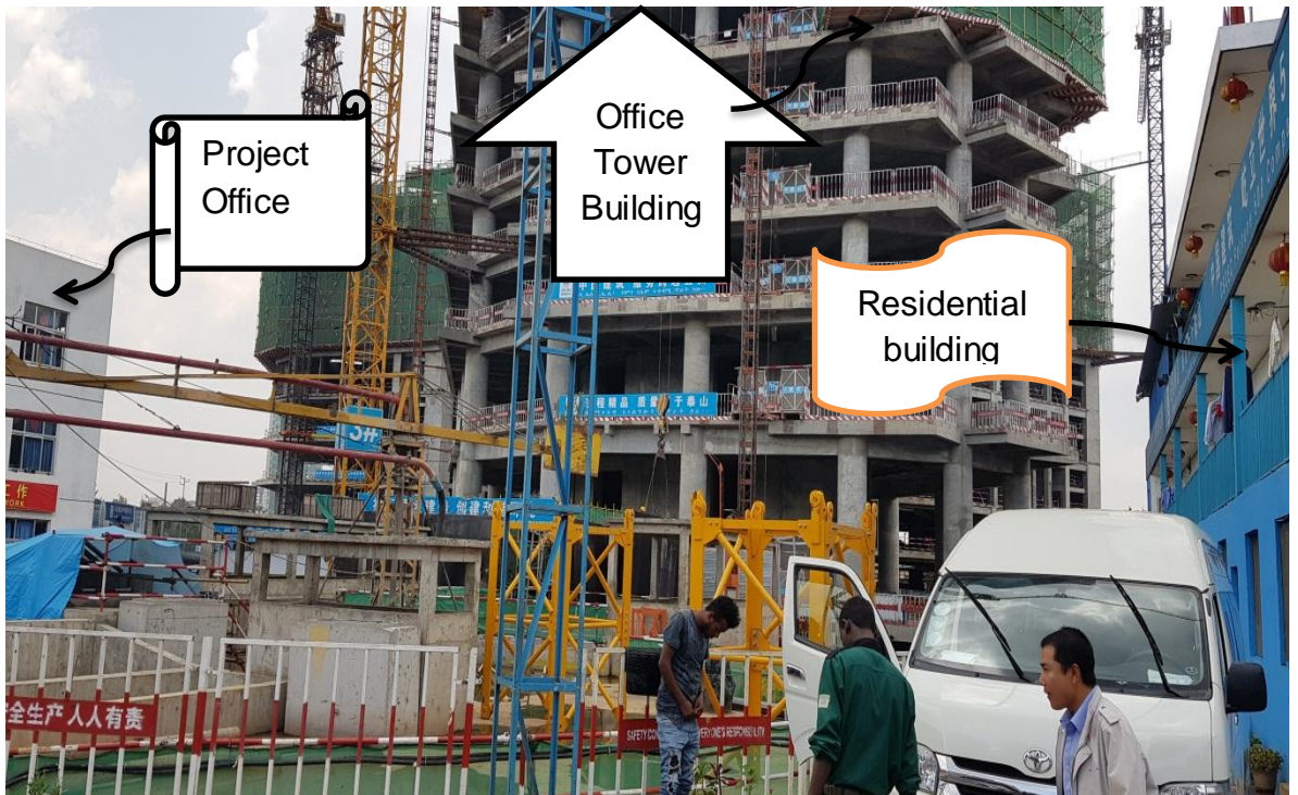
Figure 28 Contractor project office and resident building location inside the site
