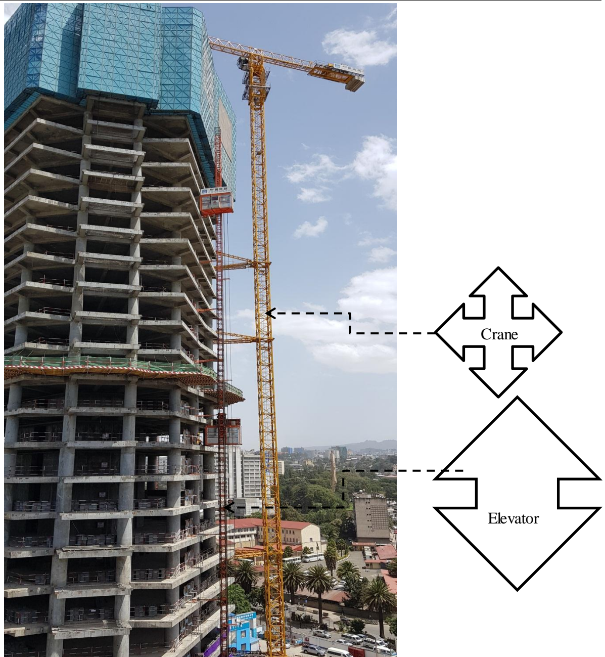
Figure 6 Tower crane and elevators
