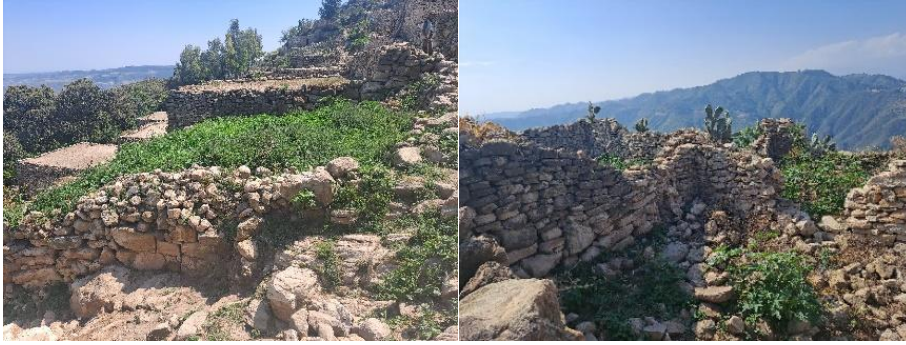
Figure 5.18 Demolished house during December observation
