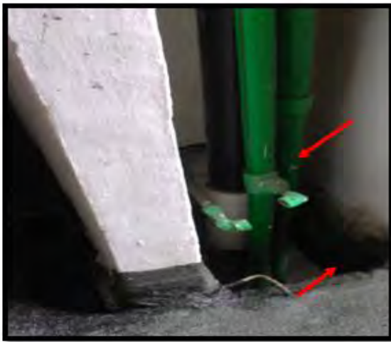
(a) uncovered floor slab along with the pipeline
