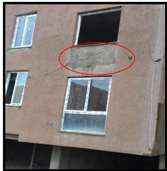
(b) plastered to fill opening along walls
