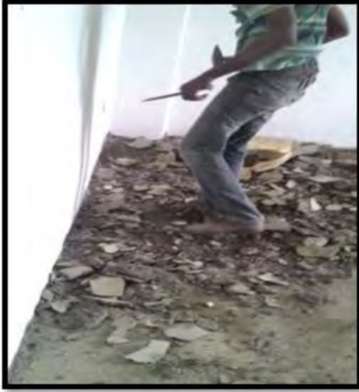
(c) Reworking on floor finish
