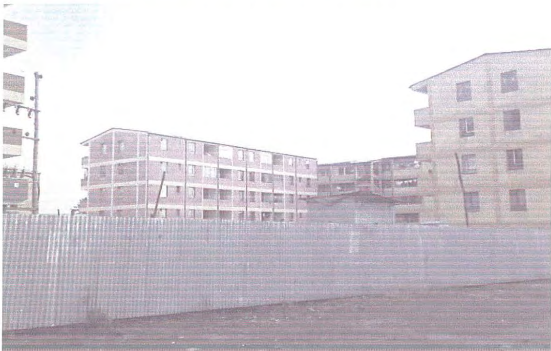
Plate.2. 34-Meda condominium site (back side) (own picture)
