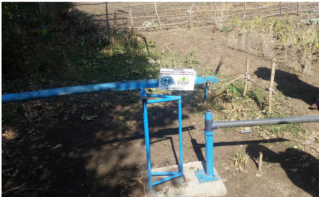
Fig 6.4 Tube well in Becho area
