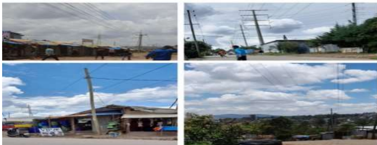
Figure 8: the high tension power lines near to commercial and residential house.
