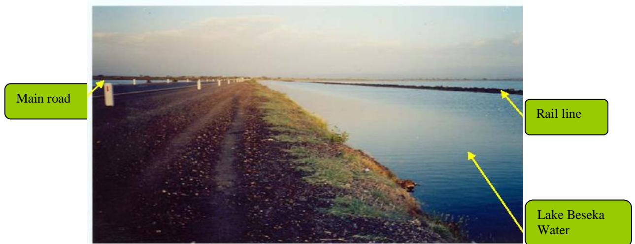
Figure 6.1. Inundation of rail line and main road by Beseka Lake (Amare, 2005)
