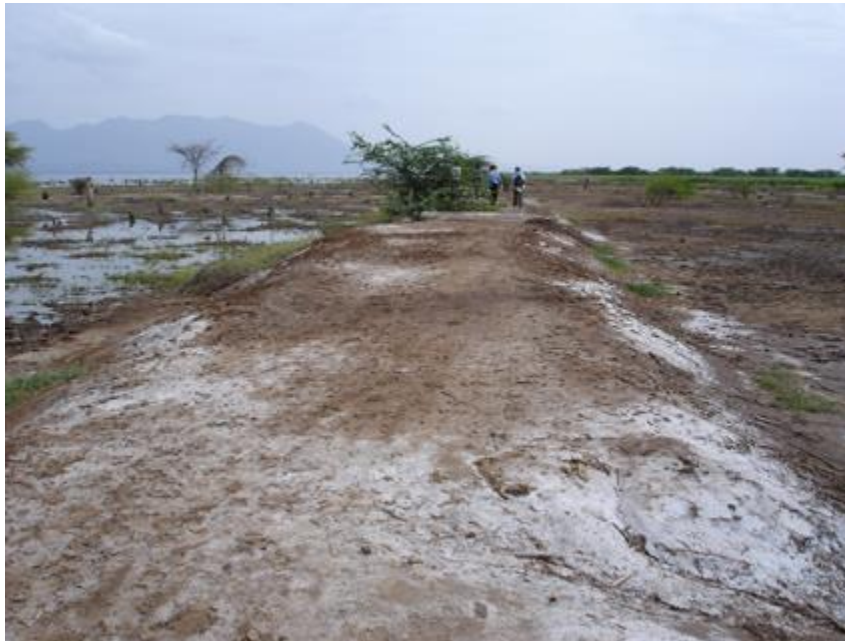
Figure 6.2- A dam built on the southern shore of Lake Beseka to prevent further damage to the Abadir sugar cane plantation (adopted from Goerner, A., 2005).
