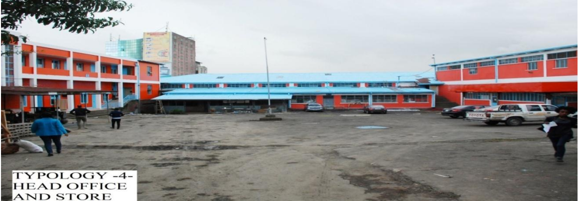
Figure 6: Partial pictures (Photo) of head office building
