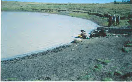
The Maja dam (constructed in 1988 EC) Unsafe water supply source for Roge- Abu Community.
