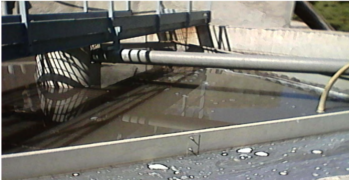
Picture 2:-Some portion of HAFPLC ETP
