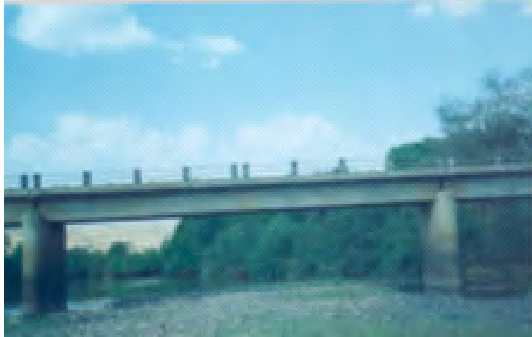
Figure 3.1 Main Gibe Bridge
