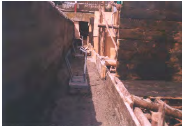
Figure 3.7 Steel Bearings of Adua Bridge
