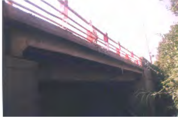
Figure 3.9 Sar Bet Bridge
