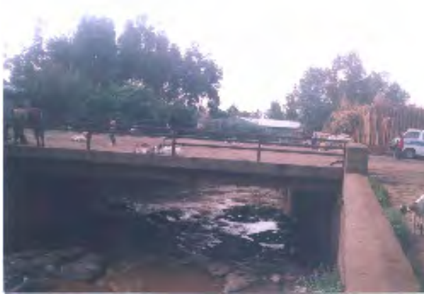
Figure 3.8 Clinic Bridge (Lideta Tsebel)
