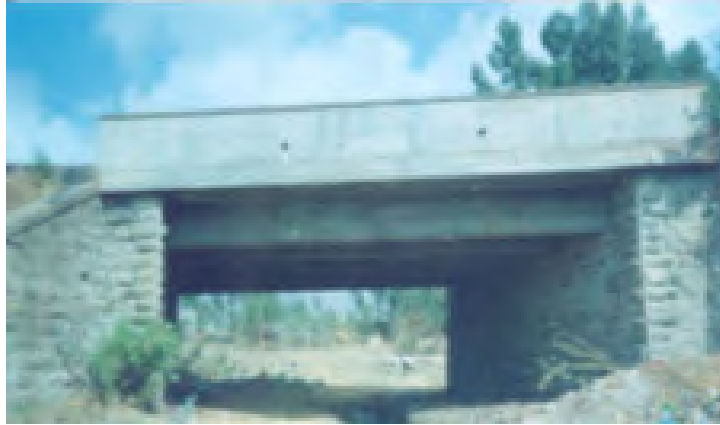
Figure 3.4 Alem Gena Bridge
