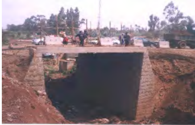
Figure 3.10 Coca Cola Bridge
