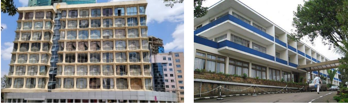
Figure 2.15: Sun Breakers on Bedelu Building (A) and Ghion Hotel (B)
