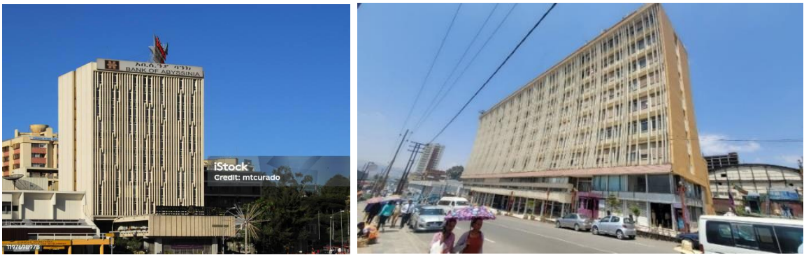
Figure 2.14: Sun Breakers on Finfinnee Building (A) and Temama Fok Building (B)
