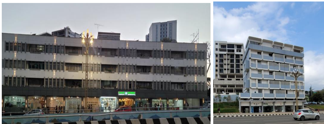
Figure 2.11: Sun Breaker styles from the Derg Era (1974–1991)
