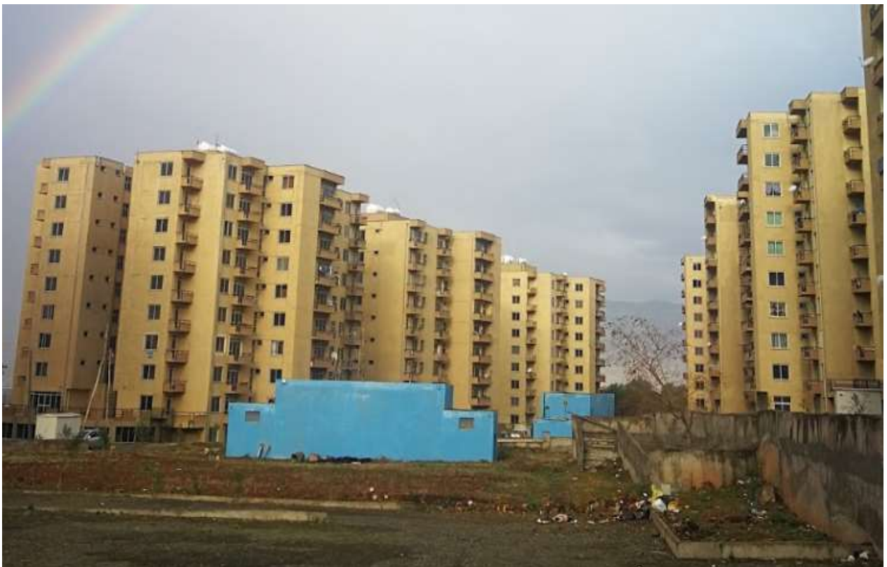
Figure 3-1 Case study building.
