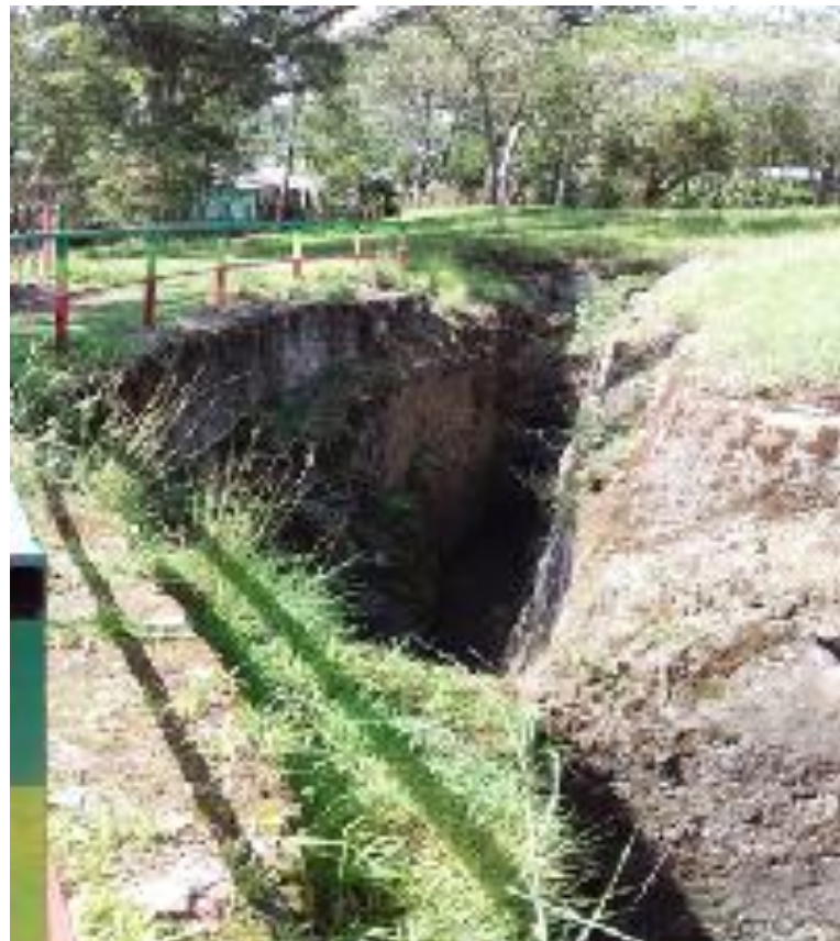
Drainage system, (Photo by the researcher June, 2020)
