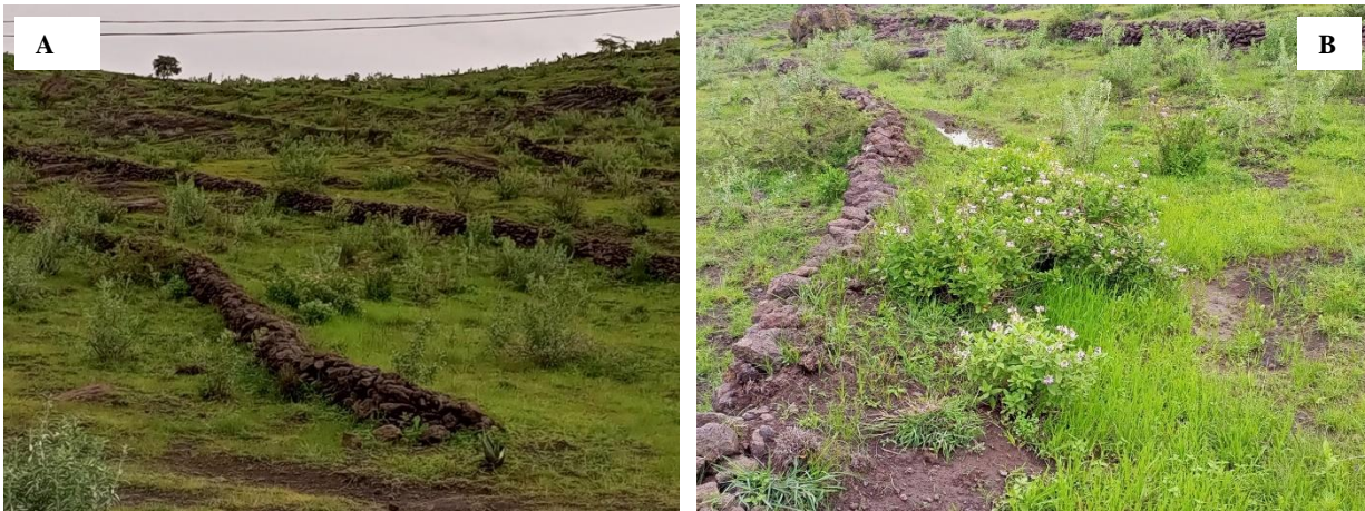
Fig. 5.10. Soil and water conservation structure on degraded shrub lands (A: Stone bund on previously degraded shrubland, and B: Soil retention and vegetation growth along the constructed stone bunds)
