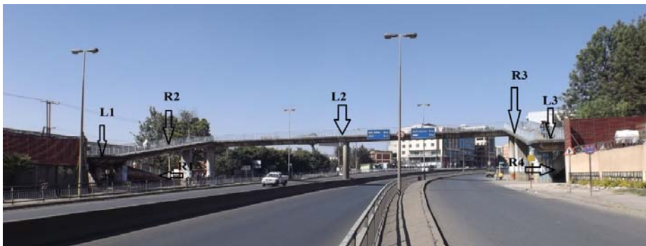
Figure 4-242 Parts of Stairway
